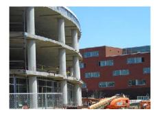
Five slabs and circular columns were poured by **concrete truck and pump**, including one slab on grade and one roof slab. Slab construction went on from the beginning of March and lasted until late May
