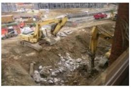
**Site work** lasted about a month and a half before excavation began for the new 25,000 SF expansion. (Excavation for new lower level auditorium above)
