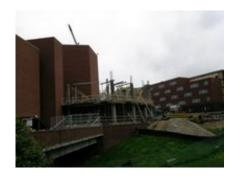
By mid December 2006, foundation work began for the new building shell. This work, along with underground drainage structures and waterproofing continued until the beginning of March, when the superstructure was cast in place.
